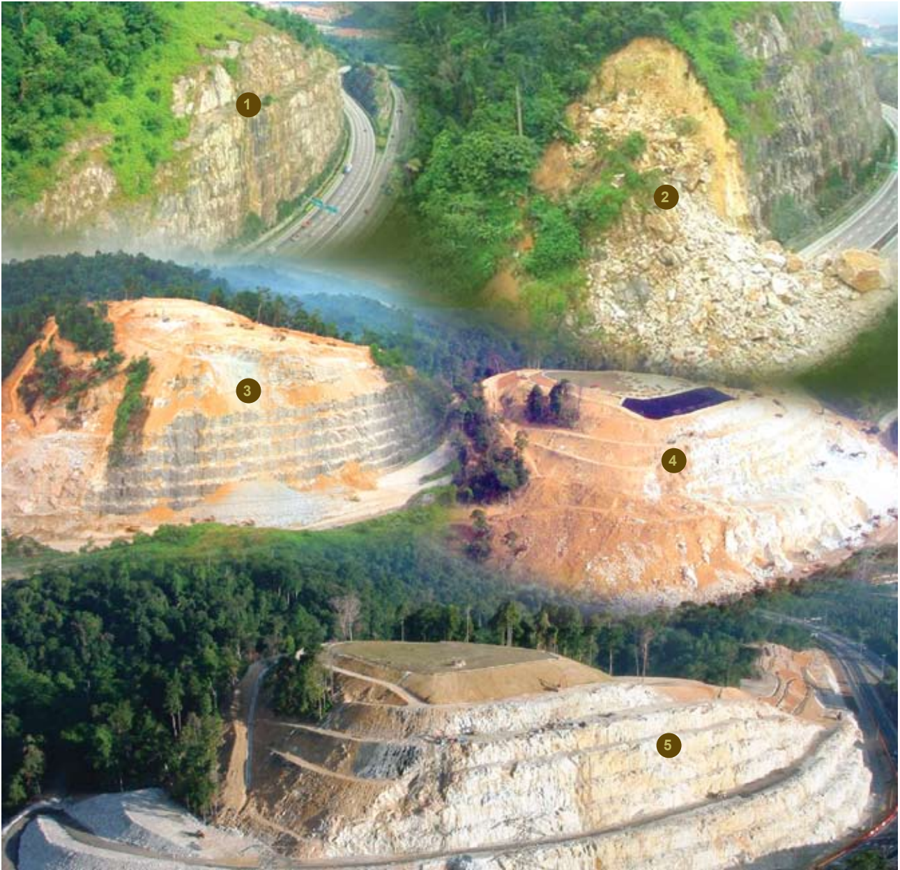
Figure 2.7: Chronology of Bukit Lanjan rockslide and repair works
